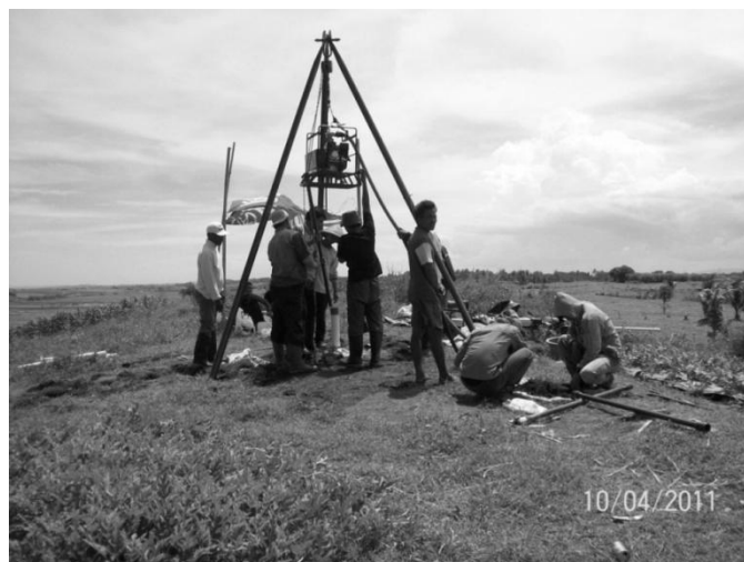
Figure 4. The power rig unit
