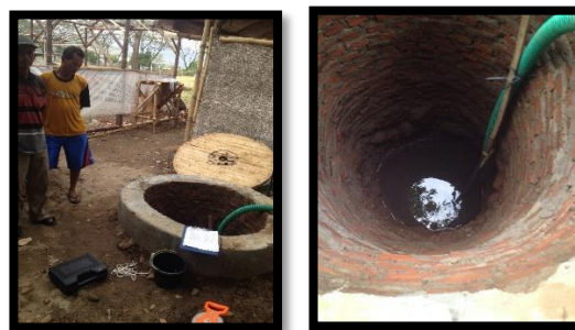
Figure 1.3 Local groundwater observation wells with moderate productivity
