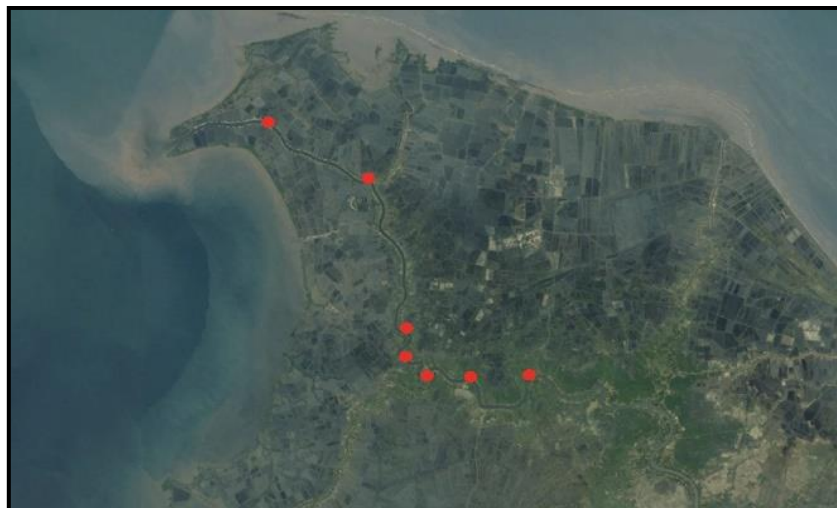
Figure 5. Embankment burst locations in Muaragembong, Bekasi Regency
